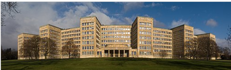
Panorama of the IG Farben Building from the south, demonstrating how the curved shape of the building's façade reduces the impact of its scale
