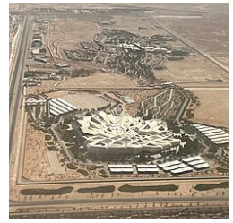
King Abdullah Petroleum Studies and Research Center in Riyadh (2017)
