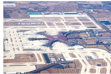
Beijing Daxing International Airport in Beijing (2019)
