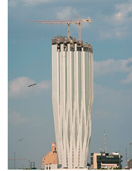
Central Bank of Iraq Tower in Baghdad (2025)
