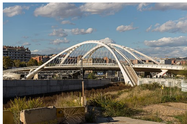
The Bac de Roda Bridge in Barcelona, Spain (1984–87)
