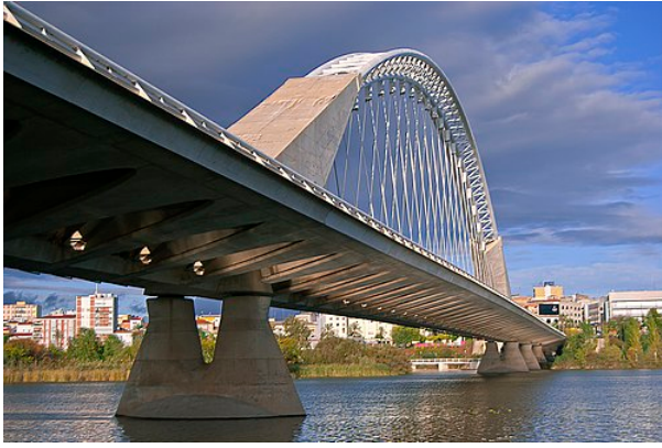
Lusitania Bridge, Mérida, Spain (1988–91)
