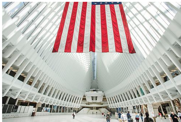
Interior of the Oculus of the World Trade Center Transportation Hub (2016)
