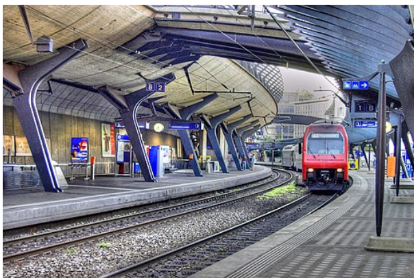
Zürich Stadelhofen railway station in Zurich, Switzerland (1983–90)
