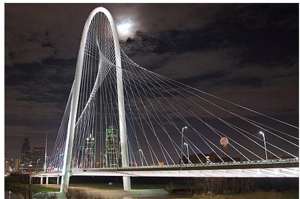
Margaret Hunt Hill Bridge in Dallas, Texas (2012)
