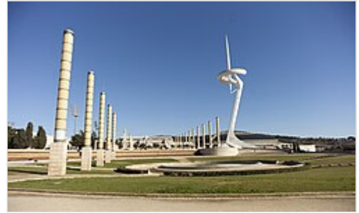
Montjuïc Communications Tower, Barcelona, Catalonia, Spain (1992)
