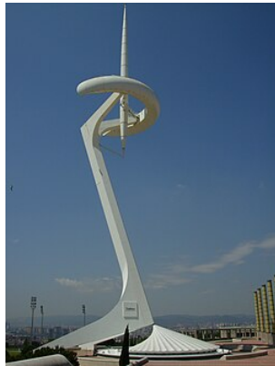
Montjuïc Communications Tower, Barcelona (1989–92)
