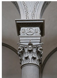
San Lorenzo, capital and elaborated impost of a column in the nave
