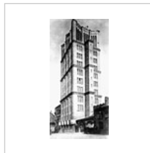
A highrise of the German Borsig company, made in the spirit of brick expressionism by Eugen Schmohl (1922–1924). It still stands in the Tegel district of Berlin .
