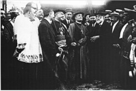
Gaudí shows the Sagrada Família to the Papal nuncio, Cardinal Francesco Ragonesi (1915). On that occasion, Monseignor Ragonesi considered Gaudí "The Dante of architecture". [41][42]
