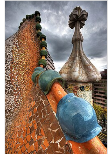
Roof architecture at Casa Batlló
