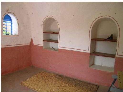
*A painted cement render on the walls and concrete floor screed*
