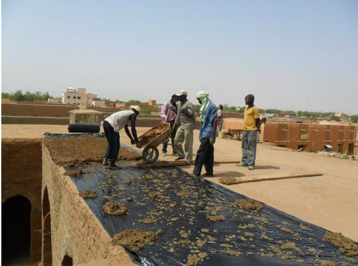
To protect the vault against rain and erosion, a tough plastic tarpaulin is laid over the roof, after it has been smoothed down and given a slight slope for draining any rain towards the gutters. The plastic tarpaulin is then itself protected with an earth mortar render of at least 5 cm thickness, using a mortar that has been enriched with waterproofing adjuvants (shea butter, other traditional 'recipes', used engine oil etc) .
