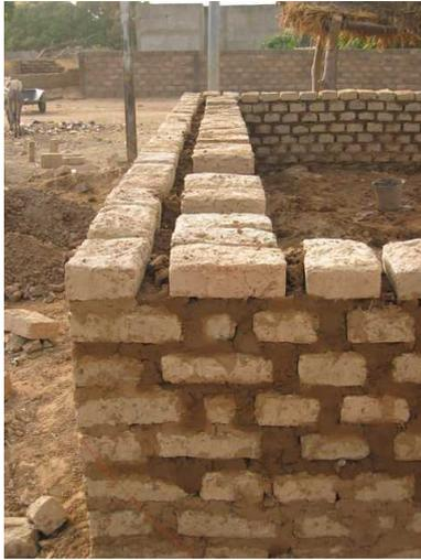
The load-bearing walls which support the vault are built of successive courses of large bricks and have a **minimum thickness of 60 cm**.
