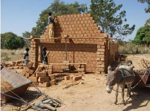
The gable walls are built with large bricks (**35 - 40 cm long**) which define the thickness of the wall. They must be built with a very slight inwards incline (of about 1 cm per metre of height).
