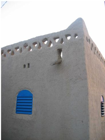
Parapets (and balustrades in the case of a flat roof terrace) should be built during the same construction phase, using mortared courses of bricks coated with the same render as the roof and walls.
