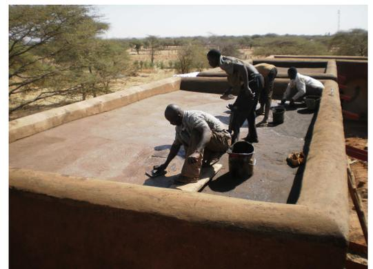
Tar-based render being applied to a roof
