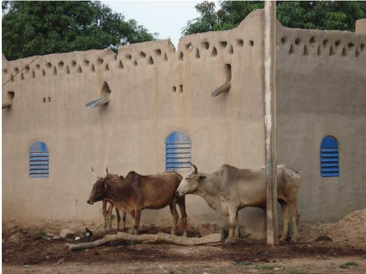
**Note:** *traditional renders are well adapted to earth architecture and have been in use for generations. The quality of the raw materials used combined with the traditional skills in their application mean that lasting results can be obtained, on condition that regular maintenance (from 1 to 4 years for exposed surfaces) is carried out.*
